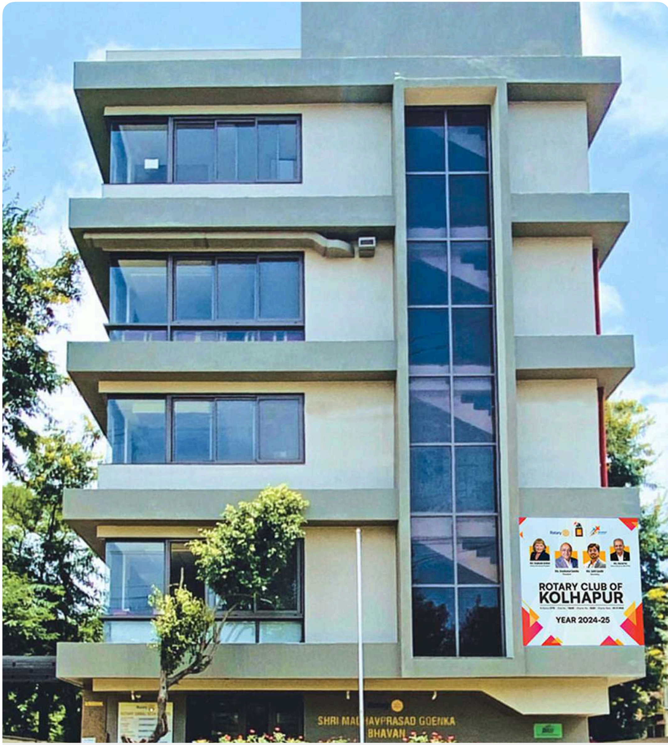
ROTARY CLUB OF KOLHAPUR'S ROTARY SAMAJ SEVA KENDRA BUILDING
